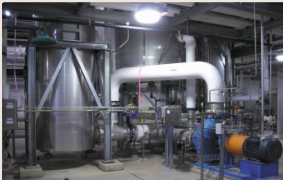
Coors Shenandoah brewhouse showing one of the external wort heaters and 1000 US Barrel combined kettle/whirlpool. The large pump right of centre carries out the circulation for heating wort to boiling point but is sized for the much bigger duty of casting through wort cooling to the fermenters.
