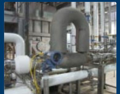
An Emerson Micromotion coriolis effect in line density meter checks gravity on the flow from the lauter tun.
