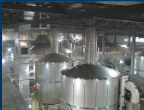
High in the roof on the way to the top of the conical FVs gives you the best view of the plant layout. You can see three coppers, two lauter tuns but the mash vessels are hidden in the distance.
